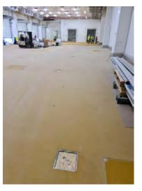
Prior to casting check that the frame protection is correctly in place. Cast the floor with the recommended fall towards the drain. Cast the floor to the desired height.
