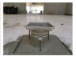
Use protection (wooden or carton board, etc.) to cover the floor drain opening. This will prevent concrete from entering inside the floor drain while pouring concrete.
