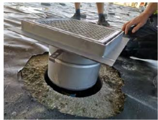
Bend out the anchor tangs at 90 ° to the drain. Adjust the drain to the right height and make sure it is level.
