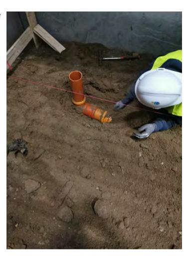
Wipe the outlet with a cloth and apply lubricant to the outlet for easy connection between stainless steel outlet and piping. Connect the floor drain outlet to the underground piping system. Make sure the connection is tight.
