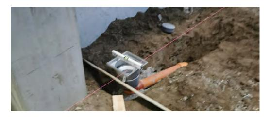
Use the levelling feet to anchor the floor drain to the floor and adjust its height. Fix the drain to make sure that it will not float up during casting. If am equipotential bond is required, connect the earth wire to an anchor tang.
