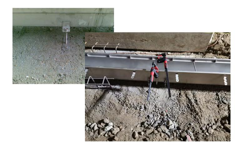
Place the channel at the required height. Use the levelling feet and height regulation nuts for that purpose. The channel always is positioned below floor level, according to the project specification.
