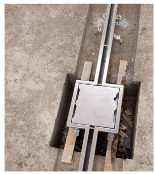
Make sure the channel is well aligned, then bolt it down to the concrete floor using the holes in the levelling feet for that purpose.
