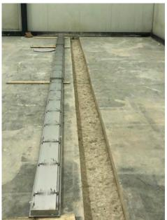
Check the channel installation height on the drawings and fix the levelling feet at the approximate final position.
