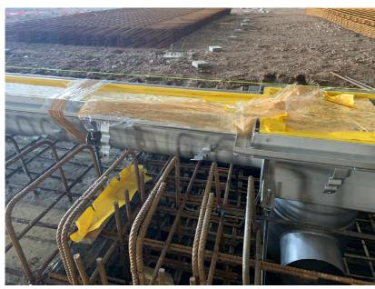
Pour concrete around the levelling feet and anchoring elements. Pour concrete up to the required level.
