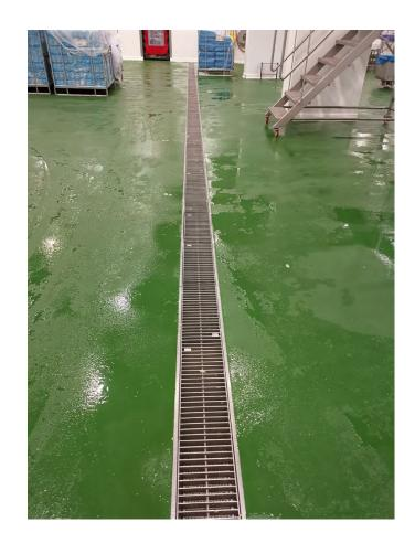
Make sure all elements are clean, free of dirt (dust, sand, concrete, etc.). Remove the timber panels and mount the stainless steel gratings.
