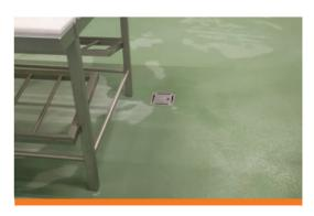
ATT manufactured more than 600 meters of stainless steel channels with plate / anti-slip mesh gratings, as well as 36 floor drains with reinforced edges:
