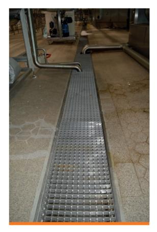
ATT manufactured more than 600 meters of stainless steel channels with plate / anti-slip mesh gratings, as well as 36 floor drains with reinforced edges:
