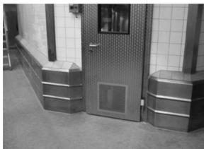
ATT offers wide range of stainless steel bollards and kerbs for commercial and industrial purposes. Elements are designed to protect warehouses stocks, production machinery, walls or to be used as separation between areas.
