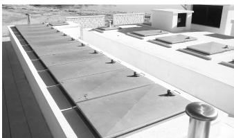
ATT offers stainless steel manhole and access covers in various shapes and sizes. Products may be equipped with accessories like: lockers, gas lifters, safety scissors, hinges, insulation, fall protection mesh, ventilation cup, ladders. Up to D load class availability.
